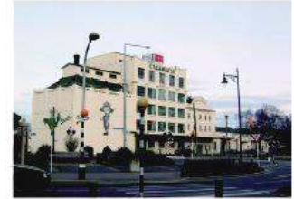
General Feedstuffs Installation - complete remodel
